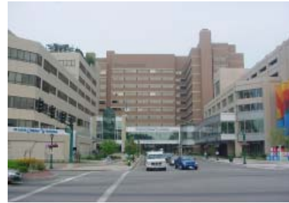
Pedestrian Bridge & Receiver Lobby
